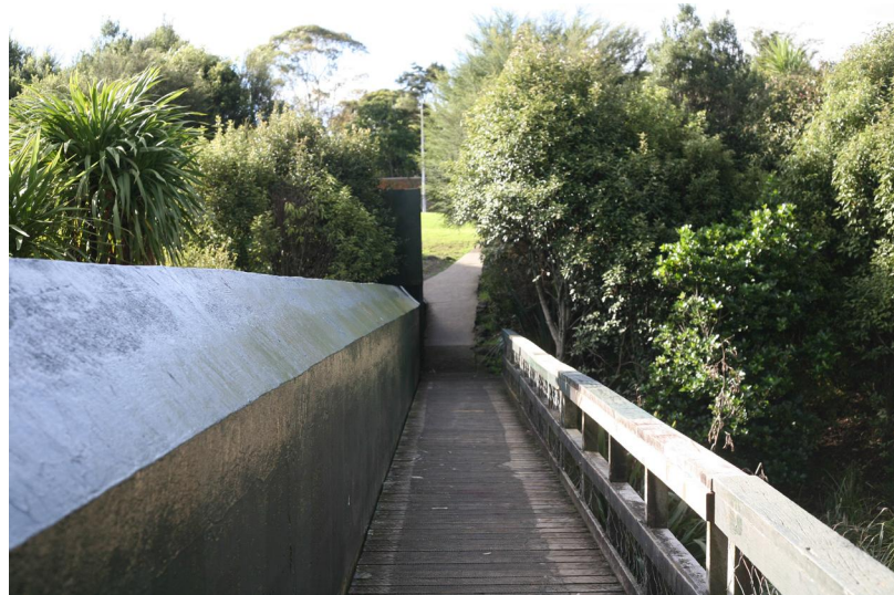
View from Pedestrian Bridge
